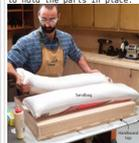
3. Glue the torsion box on your tablesaw. The surface of the saw virtually guarantees a flat top. Place the hardboard face down on the saw, spread a uniform film of glue on the hardboard and lay the torsion box on it. Weight the sandwich with sandbags.
